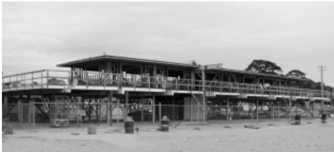
O'Neill Building under reconstruction - January 2004
